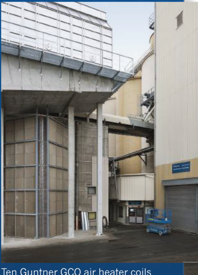
Ten Guntner GCO air heater coils (still without casing in the image) produce hot air for the kiln.
