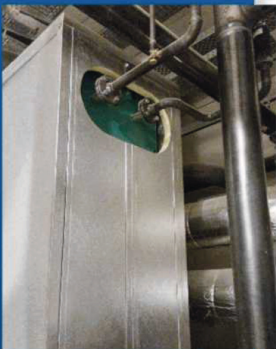
The German heating system regulation stipulates that plate heat exchangers are to be jacketed.
