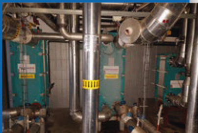
▲ thermowave TL 250 TCGL, TL 500 TCGL and TL 850 KCIL plate heat exchangers form the interface in each case between the circuits for ammonia and green beer.
